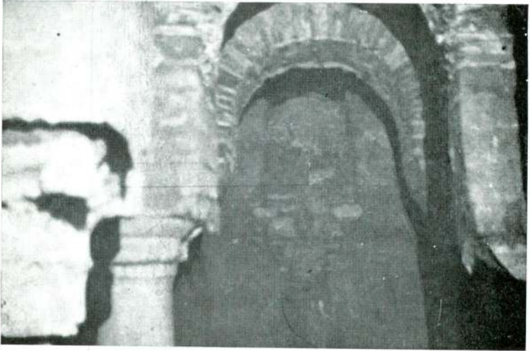
Res. 28 — Sarnıca vaktiyle ışık veren pencere yeri. Fig. 28 — Window opening which formerly gave light to the cistern.
