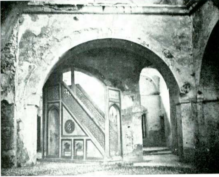
Res. 9 — Merkezi kubbeye mesned teşkil eden kemer ve pilpayeler. Fig. 9 — Piers and arches supporting the central dome.
