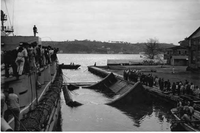
Left: The portside caisson is hauled into place on 23 February 1915.
