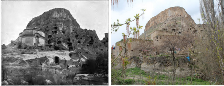
Fig. 2: On the left, the remains of Ak Kilise in 1908 (Rott, 1908); on the right, the possible location of Ak Kilise in 2019, no. 1 on the topographical scanning (author)
