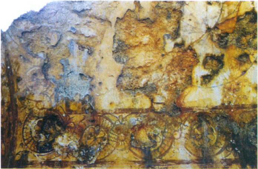
Fig.18 - The motive decorated with interlocking sparse circles surrounded vault.
