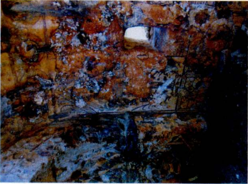
Fig.10 - The wall paintings on the apse and south wall.
