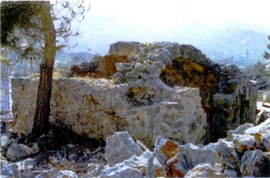
Fig.1 - External view of the chapel (from north-west)
