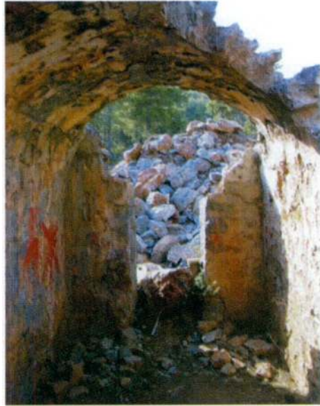
Fig.3 - Internal view (from east to west)
