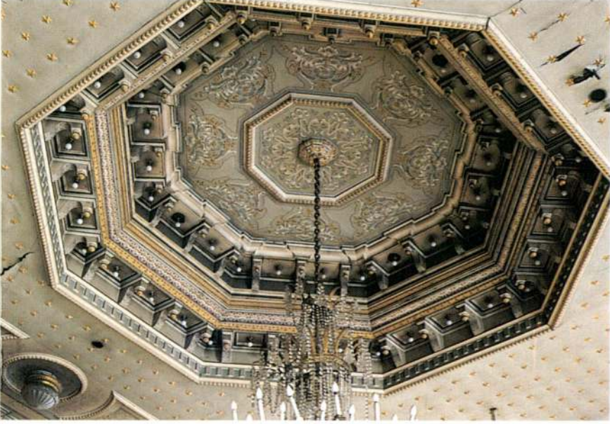
Res. 30 – Ahşap tavan - Merkezde yalancı kubbe. Wooden ceiling - Pseudo cupola at the center
