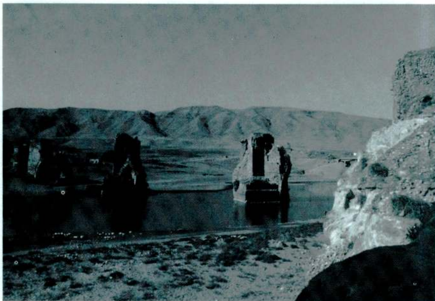
Fig. 13 — Hasan Keyf bridge.
