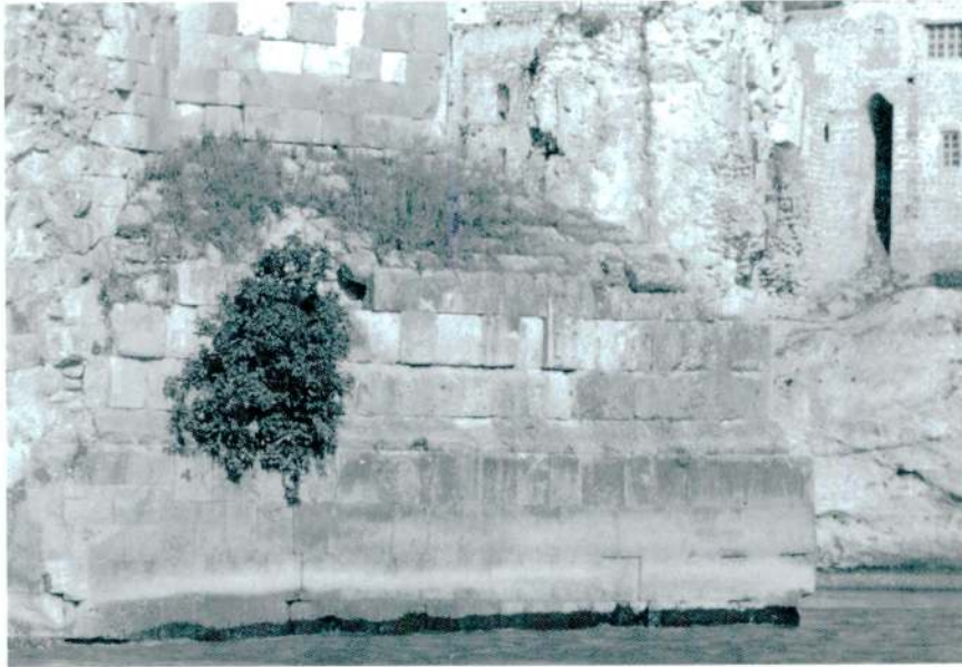
Fig. 16 — Hasan Keyf bridge.
