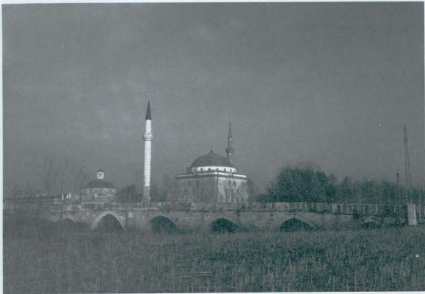
Fig. 24 — Yeni İmaret (Bayezıt) bridge.
