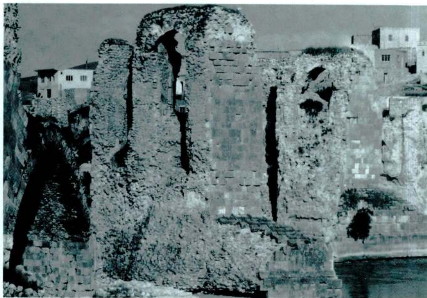
Fig. 14 — Hasan Keyf bridge.
