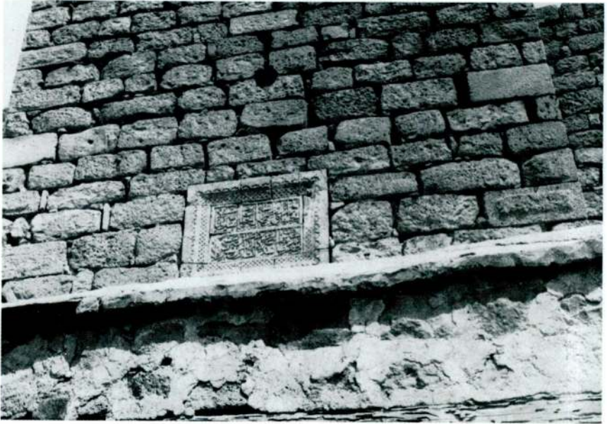
Fig. 3 — The inscription of a fountain known as Alba - Taş by the inhabitants of Diyarbakır city. The fountain is by the walls of Inner Fortress and the inscription is on the wall above the fountain.
